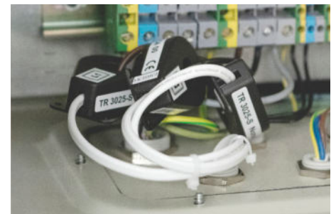
The enclosed current sensors are placed on the input phase conductors and measure the amount of current.
